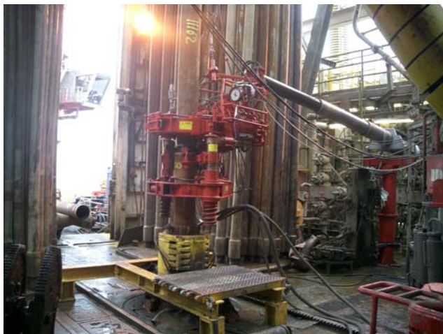
Figure 12. Snubbing slips in use when making up the liner
